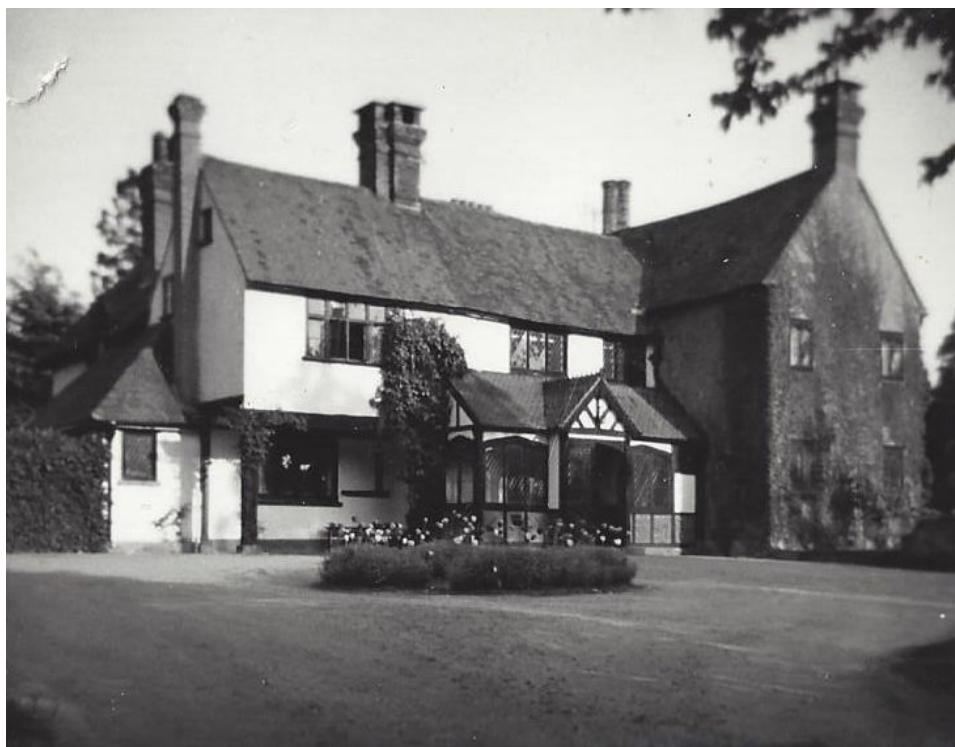
Rear of the house ©Jenkinson 2000
